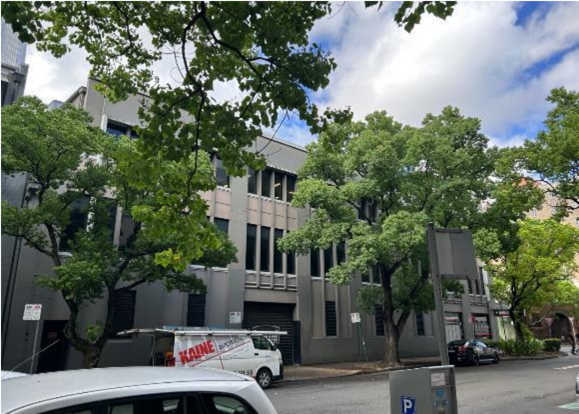
Figure 5: Existing north facade of site viewed from across Smail Street, facing southwest
