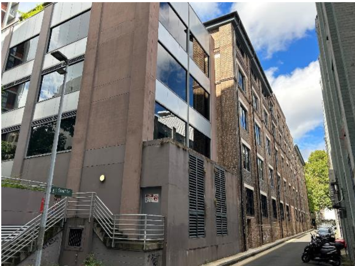
Figure 6: Neighbouring educational facility across Smail Lane
