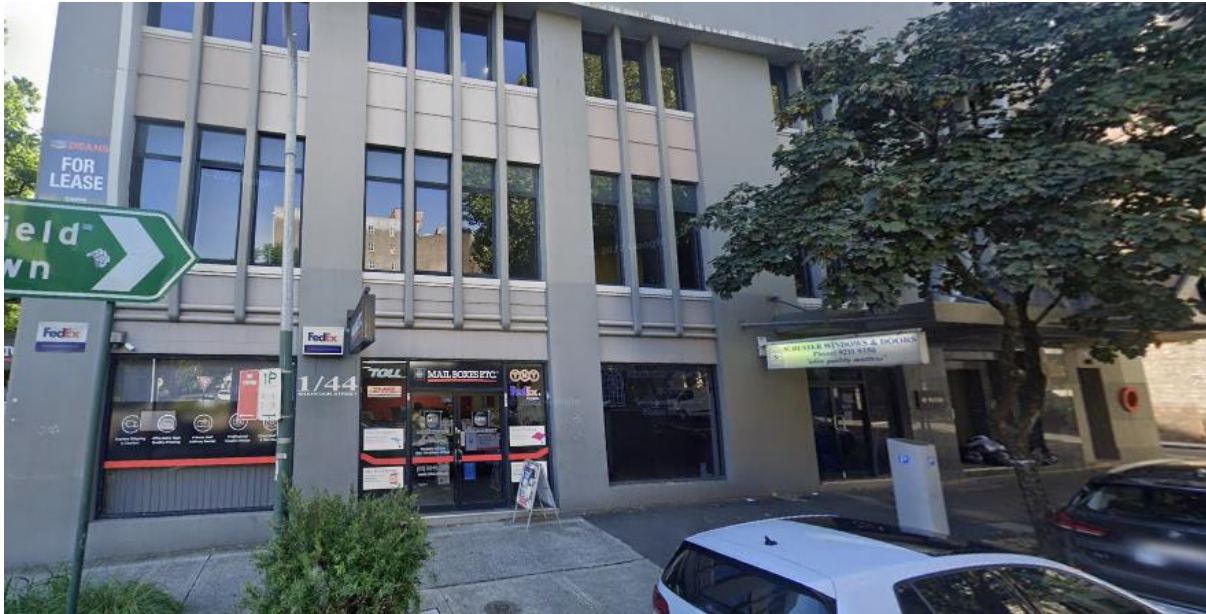
Figure 25: Image of the Mountain Street façade of the site. The horizontal and vertical trim are shown above the existing street level glazing.
