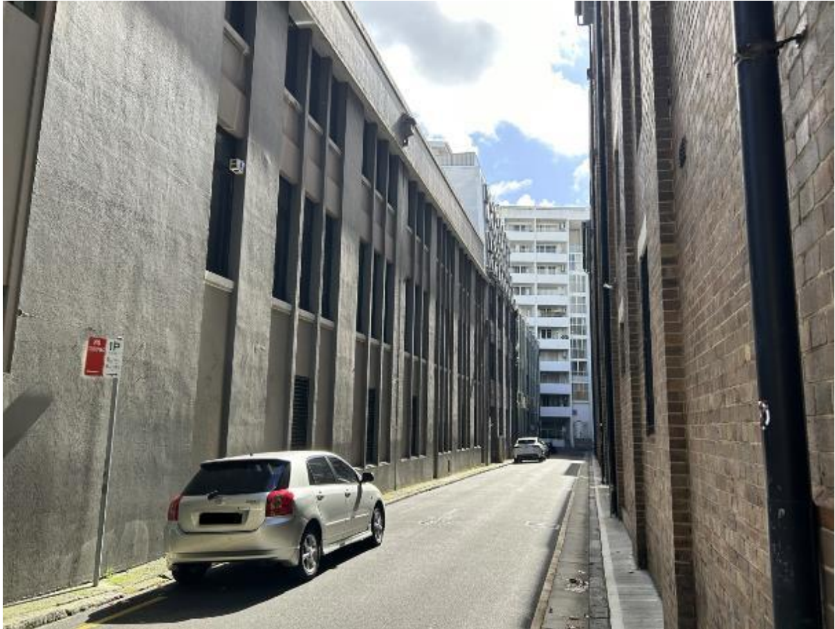
Figure 4: Site (left) viewed from Smail Lane, looking east
